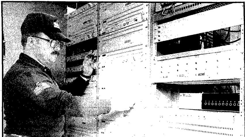
MANAGER OF THE Wayne Jones Intercable office, Bill Dennis, makes some adjustments at the station southwest of Wayne.
